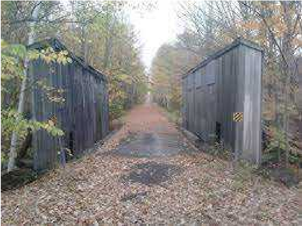
Howe Pony Truss Bridge
