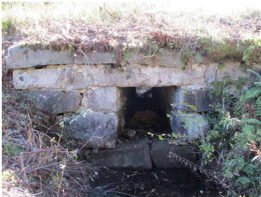
Stone culvert under the old railway bed is still in excellent condition. The railway bed is south of the Dolly Copp Wetland and also within a transmission line ROW.
